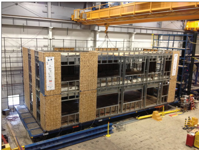
(a) CFS-NEES Phase 1 Building
