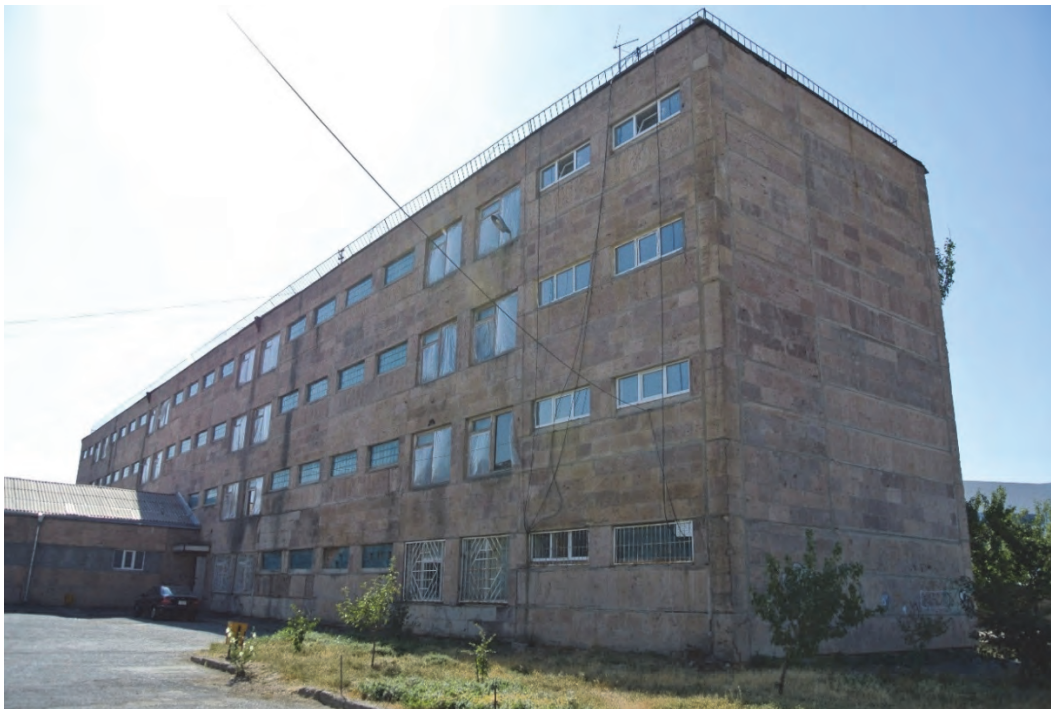
Figure 4-11 Typical four-story Typology D-2 classroom building.
