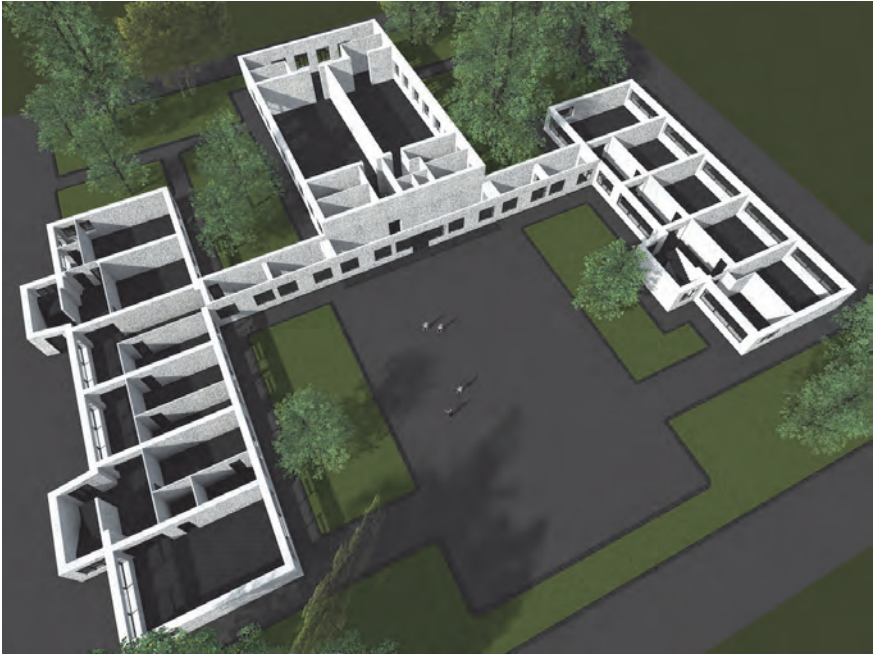
Figure 2-3 Illustration of typical school complex with multiple independent buildings, connected by corridor structures, and separated by anti-seismic joints (from EEC et al., 2015).
