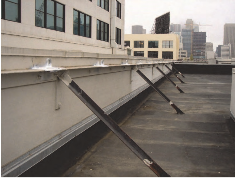
Figure 6-4 Example of parapet bracing (FEMA, 2012).
