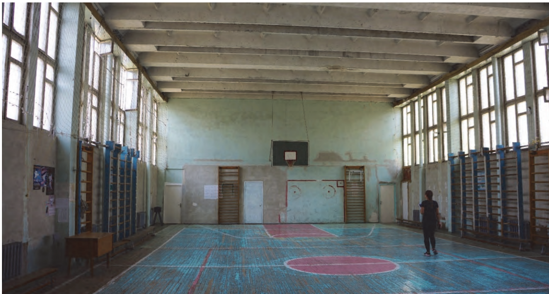
Figure 4-8 Typical Typology D-1 gymnasium building.
