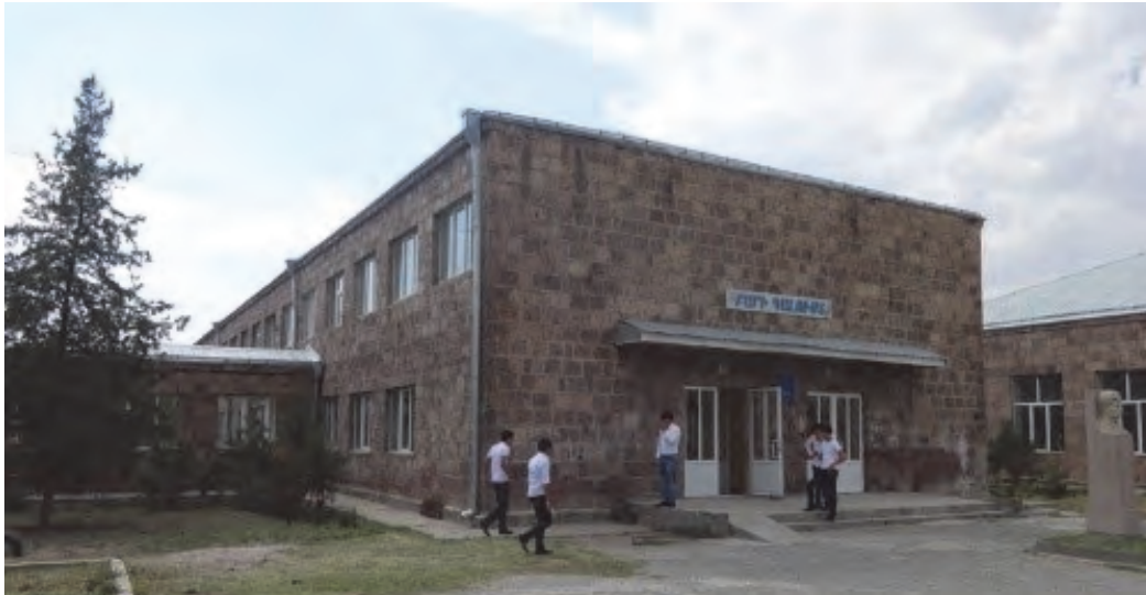
Figure 4-3 Typical two-story Typology A classroom building.
