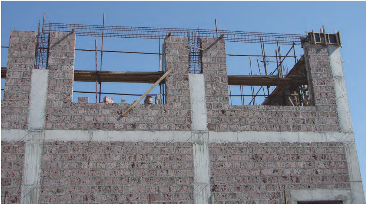
Figure 2-1 Cast-in-place reinforced concrete frame and masonry infill for a new gymnasium building under construction in Yerevan in 2016.
