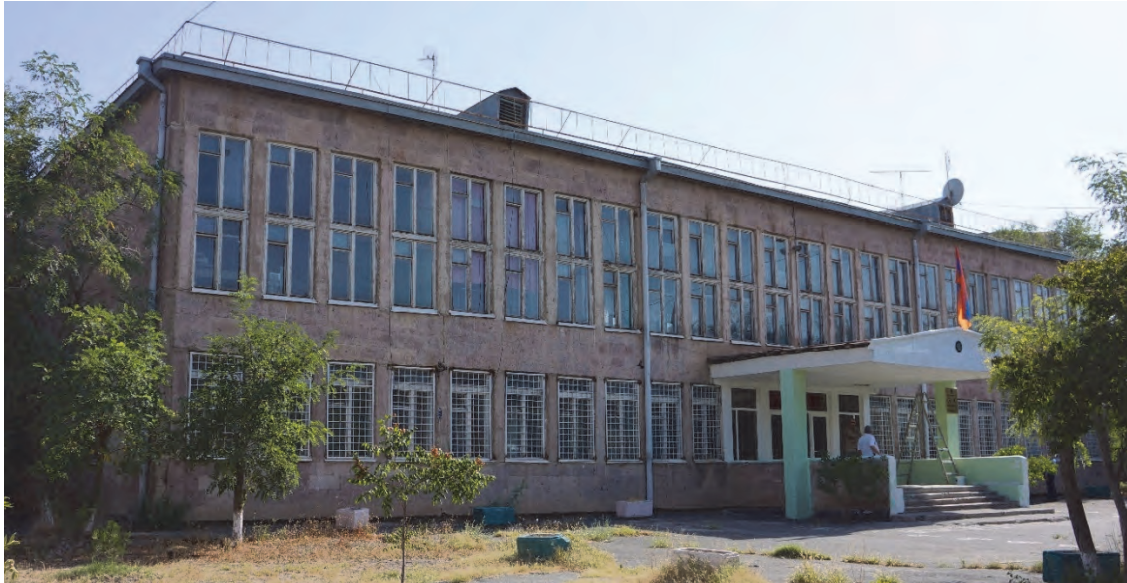
Figure 4-7 Typical two-story Typology D-1 classroom building.
